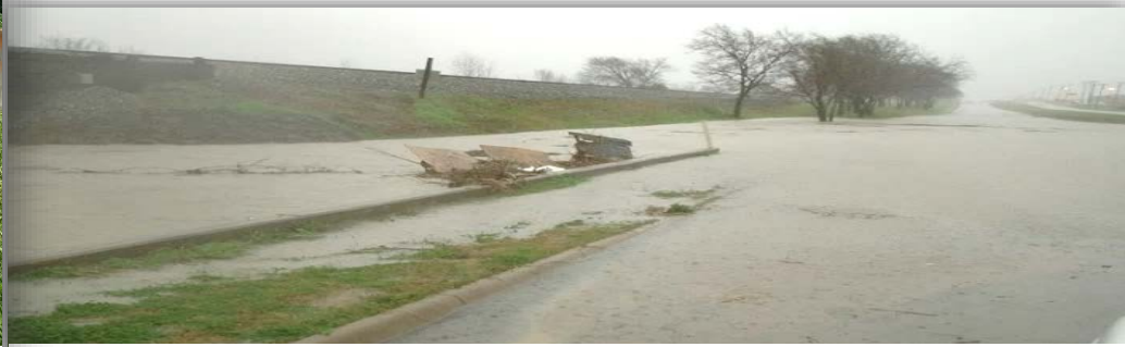
Flooding of US-78
