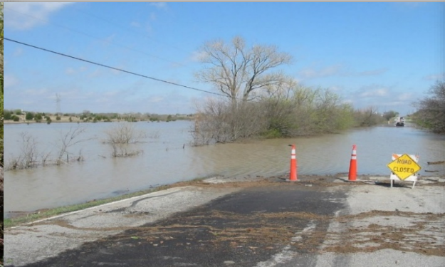
Flooding on Merritt Road
