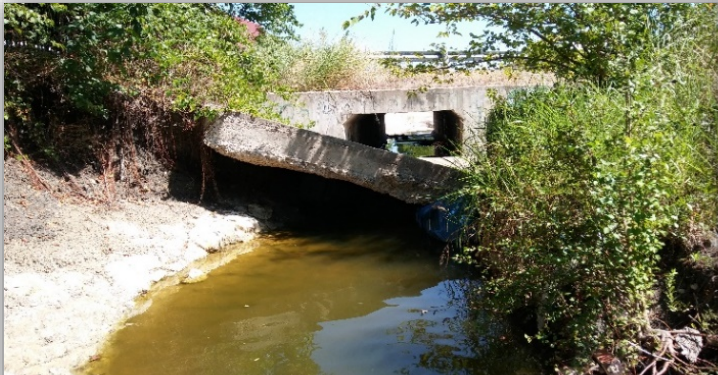
Headwall at Ingram and Dewitt Road
