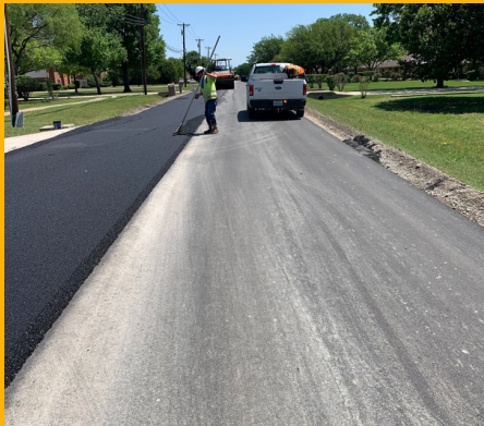
Ingram and Blackburn Asphalt Overlay 2023
