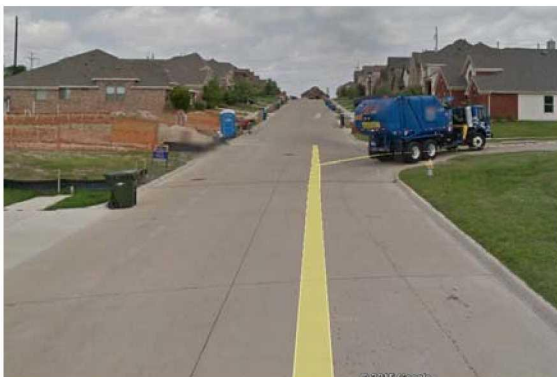
View looking to the West (up the hill)
