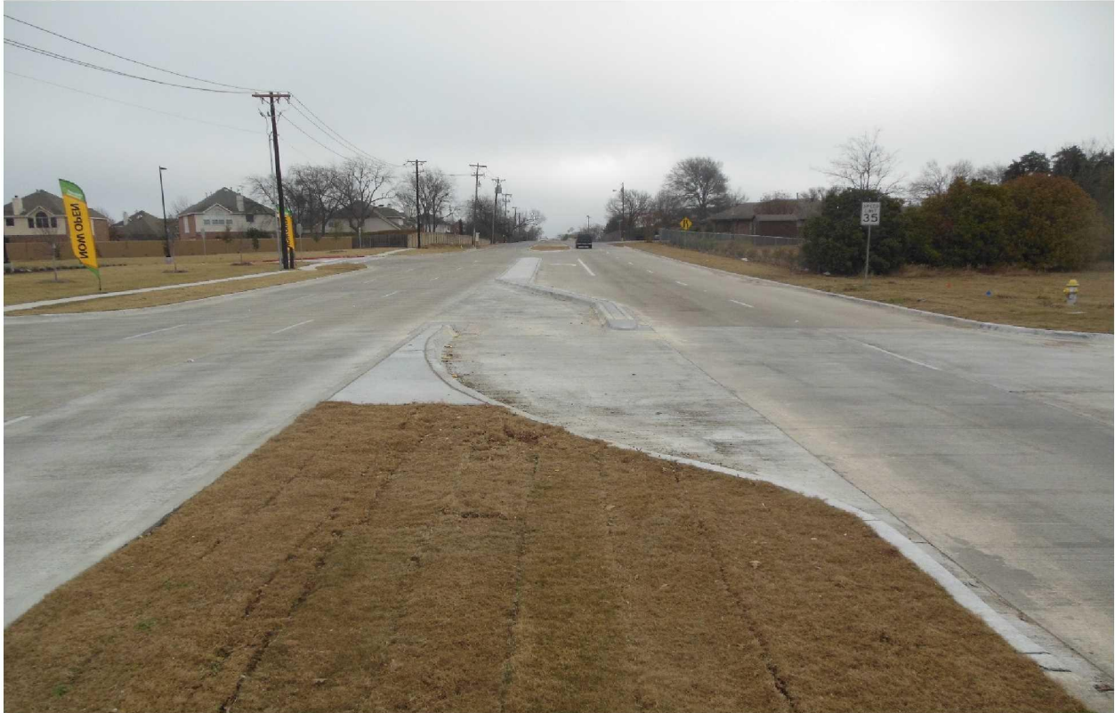
Looking to the east on Blackburn Road
