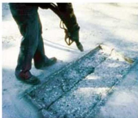
Cut out partial depth of concrete
