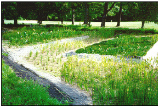
Newly Constructed Shallow Wetland
