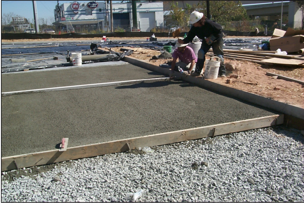
Figure 25.2 Porous Concrete System Installation
