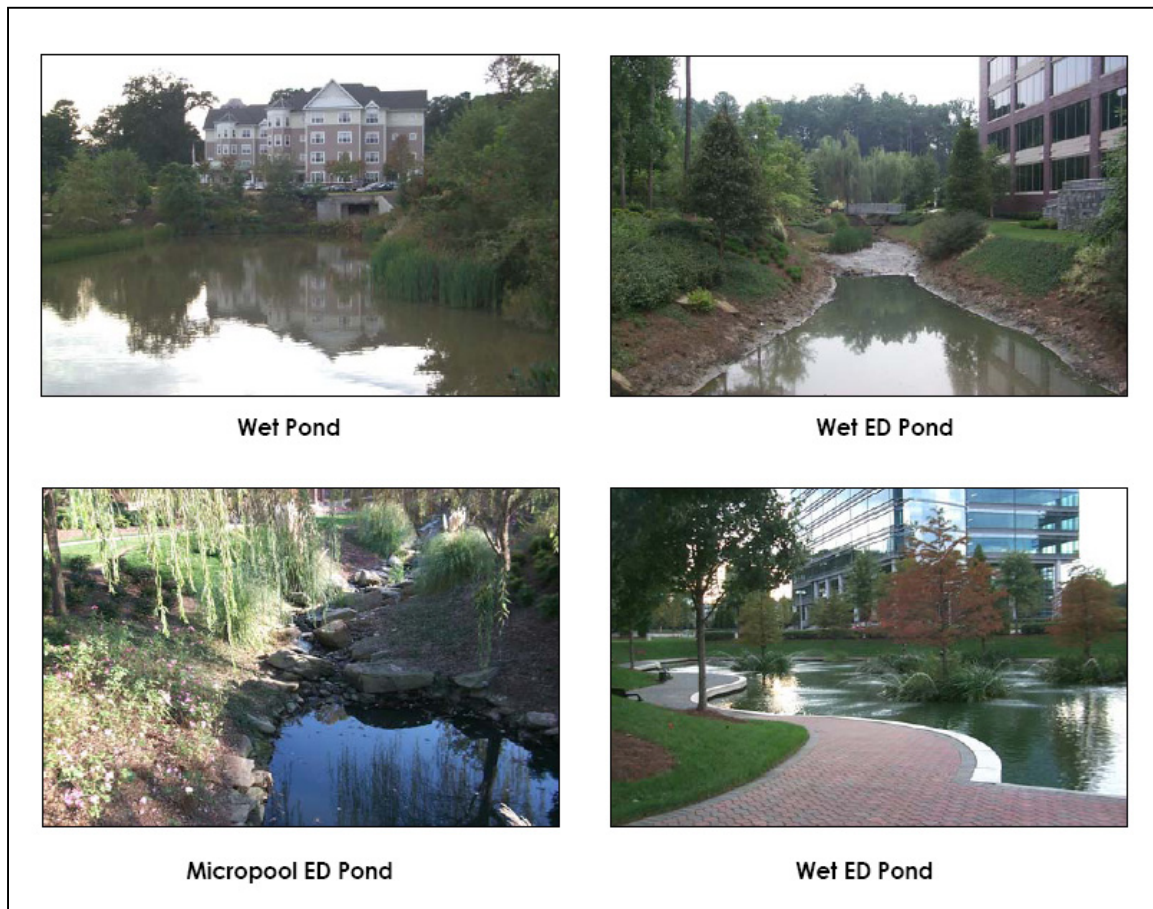
Figure 22.1 Stormwater Pond Examples
